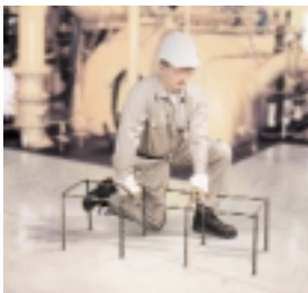
Install rebar cage
