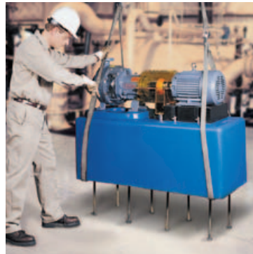
Lower Polyshield over rebar cage.
