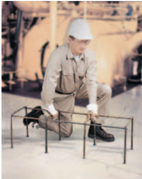
Install rebar cage.
