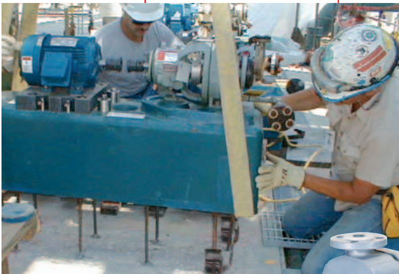
Polyshield installation at a Louisiana chemical plant
