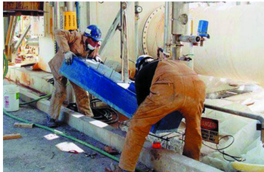
New installation of a pre-cast polymer pump base.
